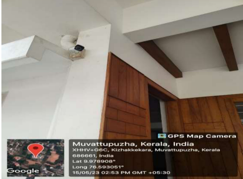
Security camera in ladies hostel
