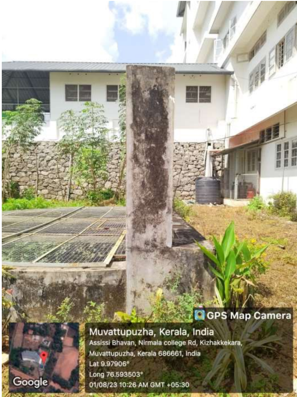
Drinking water well in hostel
